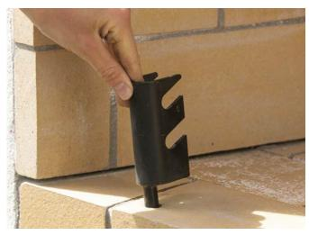
Drill 2 x 12mm diameter holes in the front row of the firebricks. Push log retainer holders in place.
