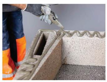
Apply the jointing adhesive on top of the first layer.
