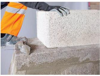
Press the first chimney block into place, checking it is in the correct position above the hole in the top plate.
