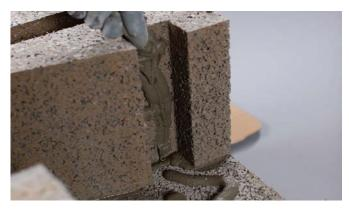
Press one side block into place and apply jointing adhesive into the slot as shown.
