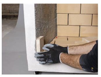
Once the bottom and rear firebricks are in place, fasten the side bricks in position using the firebrick mortar. Use a tile spacer to keep an 8mm gap.
