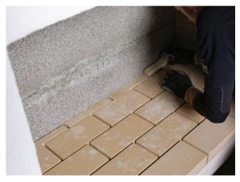
Complete the bottom layer of firebricks, then fasten the rear firebricks in place using the firebrick mortar. Use a tile spacer o keep an 8mm gap.
