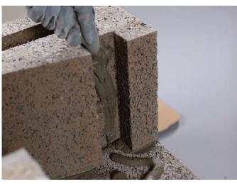
Press one side block into place and apply the jointing adhesive into the slot as shown.
