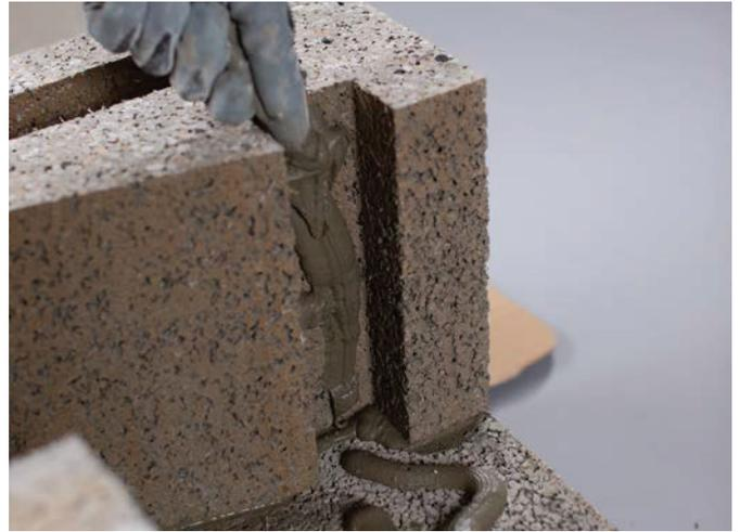
Press one side block into place and apply the jointing adhesive into the slot as shown.
