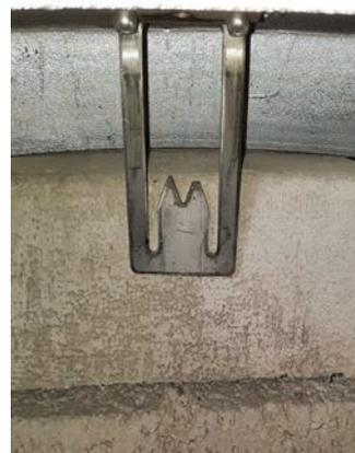
Bend the steel prongs out so the Rain Cap is a tight push fit into the concrete Top Cap.
