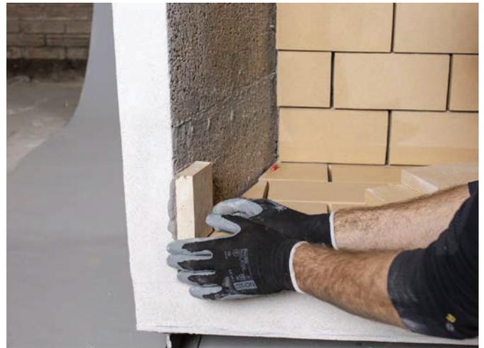
Once the bottom and rear firebricks are in place, fasten the side bricks in position using the firebrick mortar. Use a tile spacer to keep an 8mm gap.
