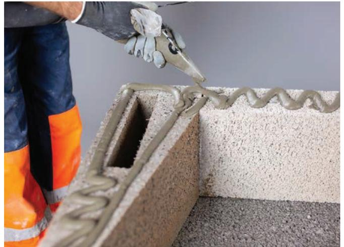
Apply the jointing adhesive on top of the first layer.
