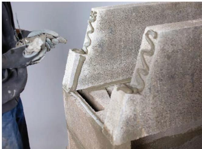
Apply jointing adhesive to the joints on the sides of the front and rear panels of the gather.
