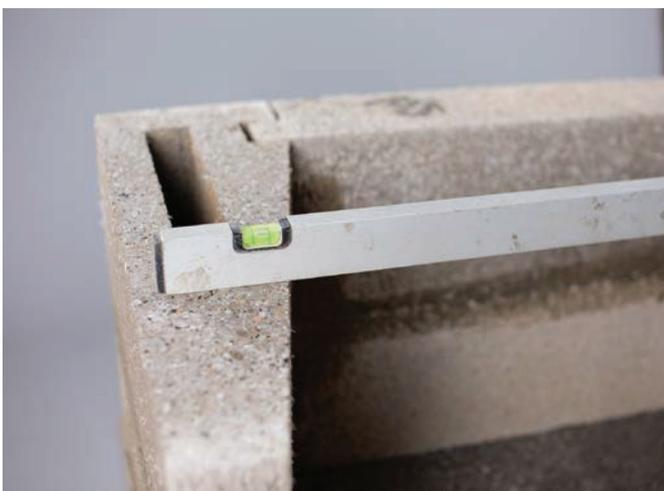
Add a further 2 layers of side blocks and back panels applying jointing adhesive between each layer and at each joint. In total there are 3 layers on top of the base plate, as per the image. (If the log storage option is not being used, then this base plate will be bedded directly on to a suitable prepared base).
