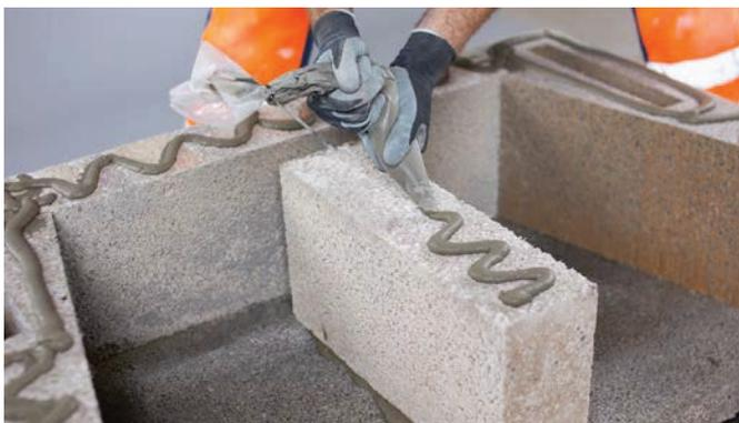
Press the middle section down on to the jointing adhesive and apply additional adhesive as shown.
