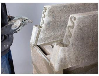
Apply jointing adhesive to the joints on the sides of the front and rear panels of the gather.
