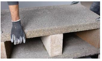
Press the base plate of the firechest down on to the log storage. Keep checking all is level and remove any excess jointing adhesive.
