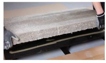
Create a suitable base. We recommend 100mm thick reinforced concrete. Bed the base plate using the supplied jointing adhesive. Check every stage is level.
