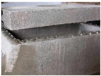
Apply jointing adhesive to the top of the gather unit and then press the top plate into position with the hole offset closer to the rear section of the gather. Ensure the top section is level. Clean off any excess mortar.
