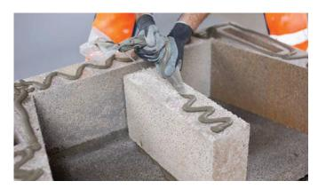
Press the middle section down on to the jointing adhesive and apply additional adhesive as shown.
