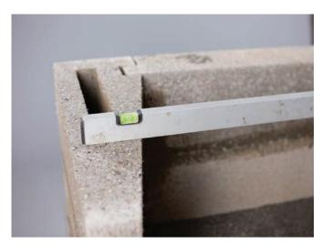
Add a further 2 layers of side blocks and back panels applying jointing adhesive between each layer and at each joint. In total there are 3 layers on top of the base plate, as per the image. (If the log storage option is not being used, then this base plate will be bedded directly on to a suitable prepared base).
