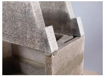
Apply jointing adhesive to the top layer and then press the front and rear sections of the gather into place.
